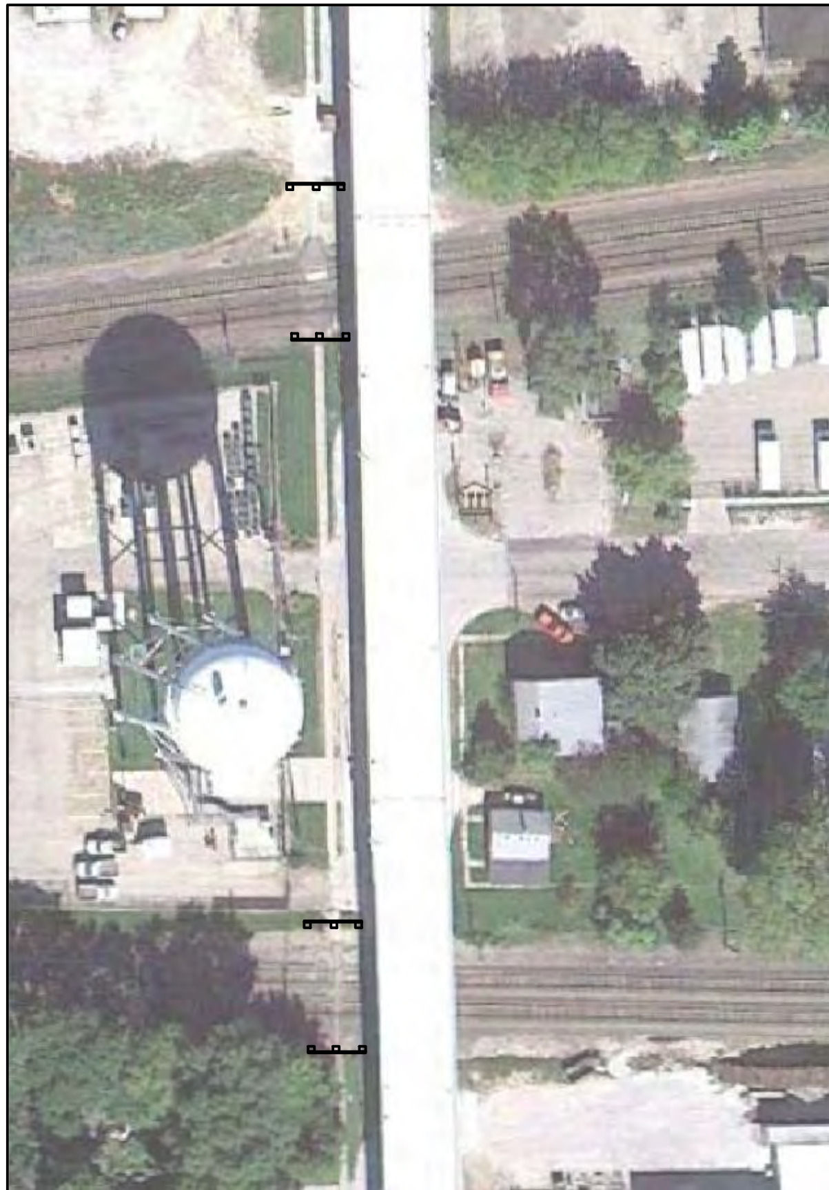
PEDESTRIAN CROSSINGS – BNSF & UPRR
