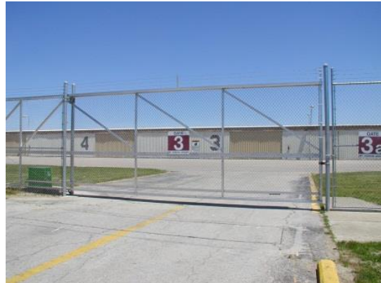
New 10-ft Perimeter Fence and Gate
