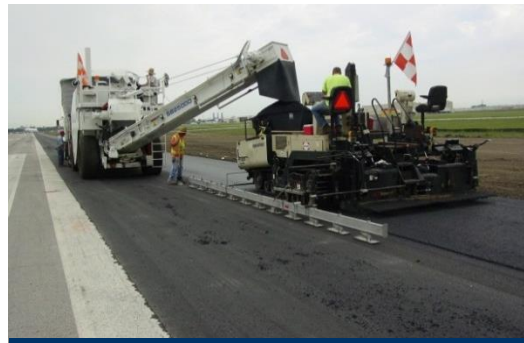
Runway 12R/30L Widening
