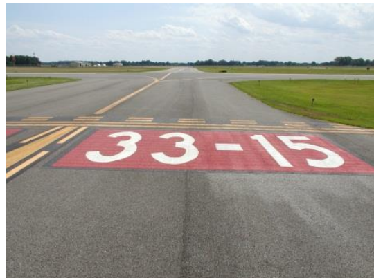
Surface Painted Holding Sign Marking
