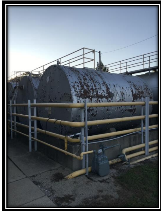
Diesel Plant Fuel Tank Removal 2020: $100,000
