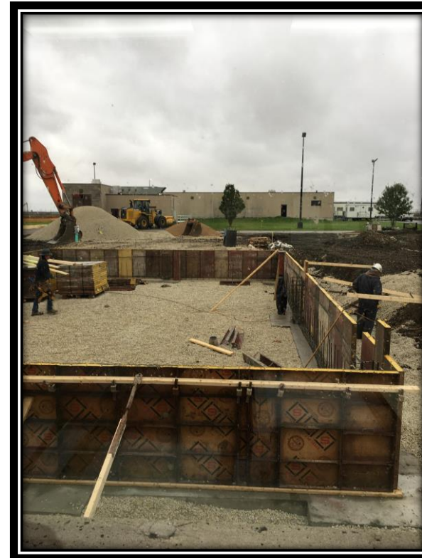
Waste Water Treatment Plant Upgrades 2020: $3,453,262 2021-2029 a total of $10,450,000
